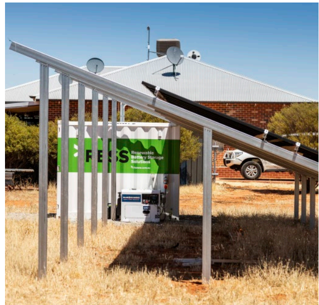
A compact diesel genset automatically provides backup power for battery charging if needed.
