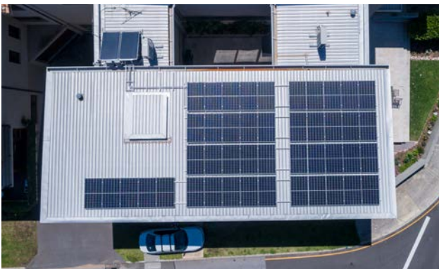
45 x 315W PV panels make up the 14kW array.
