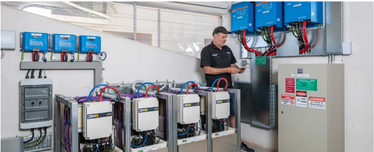
The entire BESS is monitored remotely via the Victron Remote Console feature on a smartphone or laptop.
