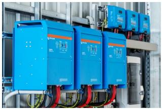
24kVA three-phase consisting 3 x 8000VA Victron Quattro Charger / Inverters
